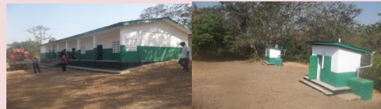
The rehabilitated WCSL primary school, Kondeya
