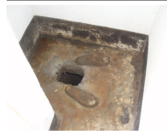
Pit Latrine at a Basic School in the Village
