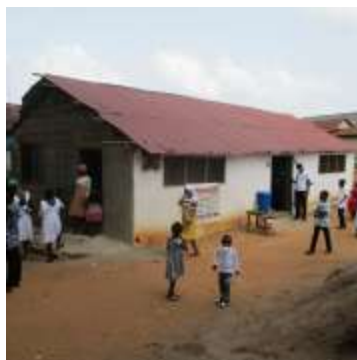
Bethel Society, Nsawam, Ghana - building erected in 2021
